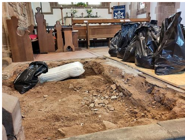
Repairs to chancel floor April 2023
